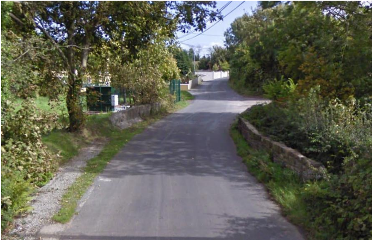
Figure 2:2: A View of The Existing Culvert from Road Level
